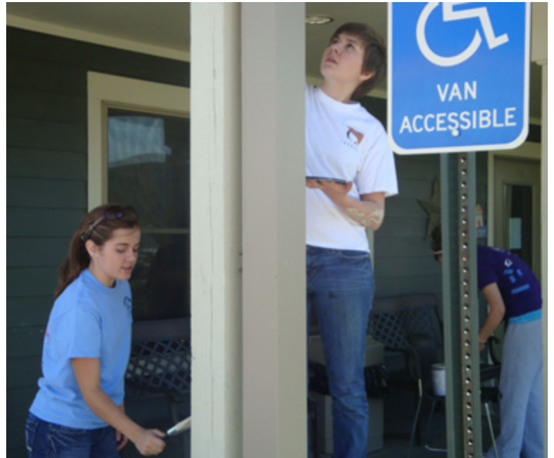
The columns on the back patio also get repainted.
